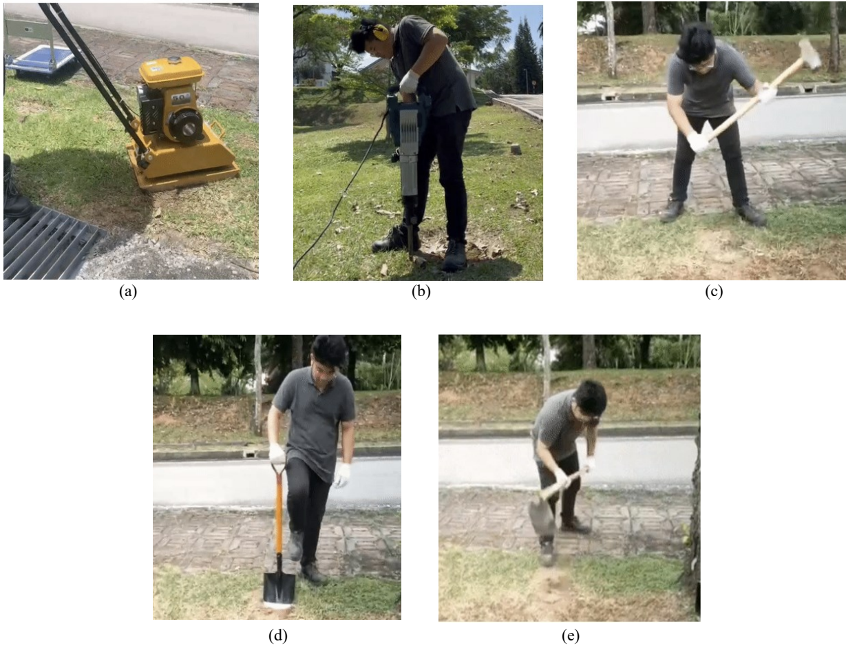
Figure 2. Simulate Disturbances to The Fiber Optic Signal using (a) Compactor, (b) Breaker, (c) Hammer, (d) Shovel, and (e) Hoe.
