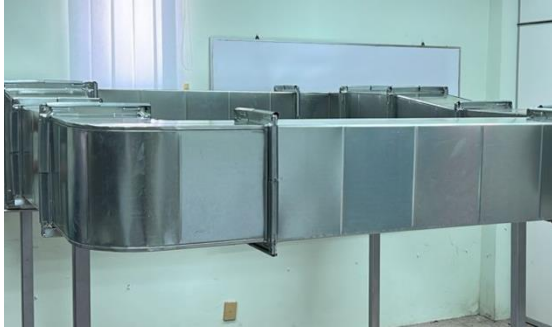
Fig. 3. HVAC ducting assembly. (Author et al. , 2025).
